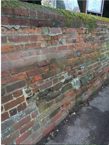
The west wall to the churchyard is in a variable condition. Some bricks have lost faces and are suffering erosion, and there are numerous open joints including to the capping bricks. The moss growth should be brushed back to expose the condition of the wall for assessment, open joints (particularly in the cappings) should be re-pointed to slow further decay and a manageable programme of maintenance of the walls put in place.
