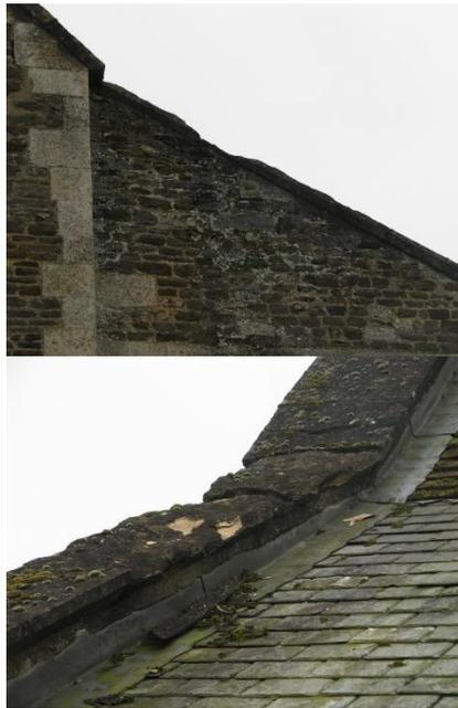
The coping to the upper section of the east parapet gable over the chapel is in poor condition and requires repair/replacement. There are signs of movement to the quoin at the eaves which requires attention and monitoring, and moss growth to sections of the wall that should be brushed clear as elsewhere.
