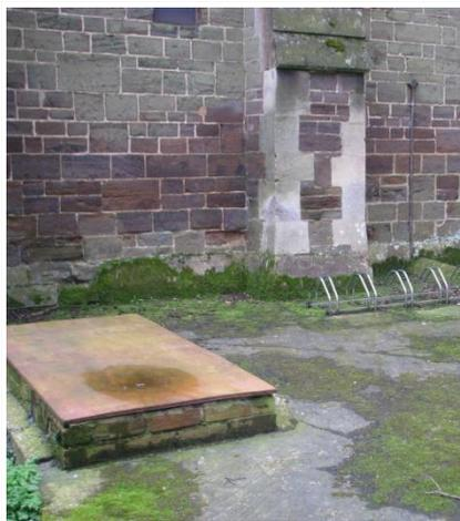
The growth of moss to the dressings and lower walls extends round to the west wall of the north aisle and over the concrete slab covering the redundant boiler room. There are signs of damp on the inside face of the wall which should continue to be monitored until the likely cause of damp penetration is addressed.
