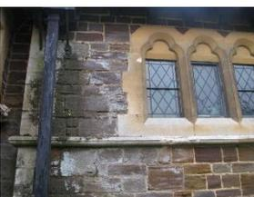
The pointing to the south side of window W8 is in poor condition most likely due to damp penetration from the adjacent downpipe and requires attention.
