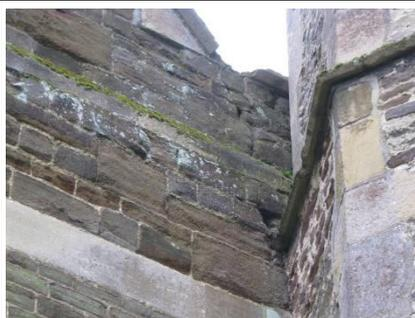
There is a broken section of coping and some stone erosion at the junction between the tower stair and North aisle west wall which require attention, together with some repointing.
