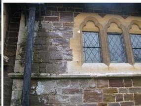
The pointing to the south side of window W8 is in poor condition most likely due to damp penetration from the adjacent downpipe and requires attention.
