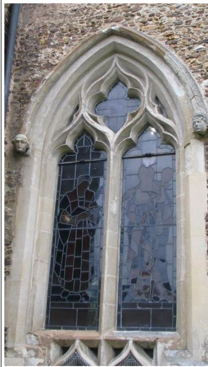
The stonework to window W3 is in a poor state in parts. The hood mould appears to have had previous render repairs which are either themselves failing or as discovered recently on the East window the render is merely masking the state of decay of the stone behind, and is the highest priority. The stone to the lower rail and jambs is in need of attention but less urgent.
