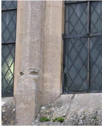
There appears to be a missing quarry to the lower corner of the north light of window W10 (at high level to the east wall of the North aisle). Closer inspection and repair is recommended. The frame in this area also requires some attention.
