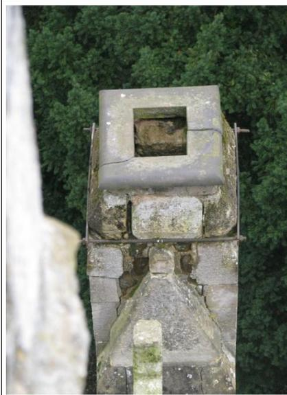
The redundant chimney is in poor condition at high level. There are signs of movement and open joints. Because of the risks associated with potentially falling masonry a close up inspection and possible temporary supports installed is recommended to be carried out as soon as practicable ahead of more permanent repairs.
