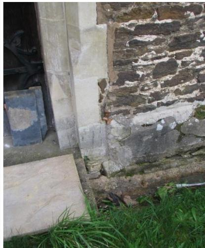
The cementitious render to the base of part of the South Chancel wall is in poor condition in parts and should be removed and the underlying stonework made good.
