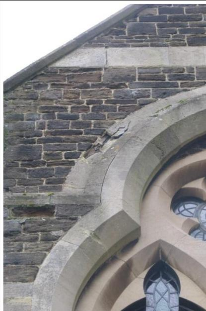
There is no hood moulding to window W15. There instead appears to be a rendered fillet over eroded stone. This render has failed to the upper north side of the window and requires repair or stone replacement.
